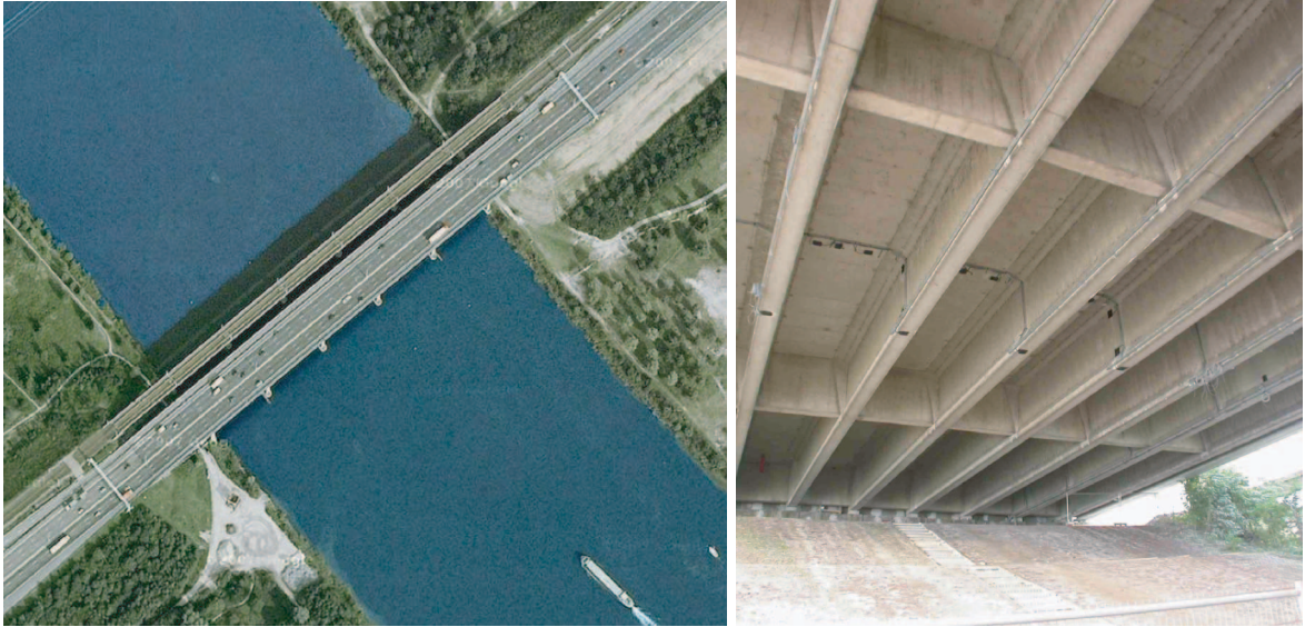
Figure 1: (left) Aerial picture of the situation of the Hollandse Brug, which connects the ‘island’ Flevoland to the province Noord-Holland, and the adjacent railway bridge. (right) Some of the sensors attached to the underside of the bridge.
